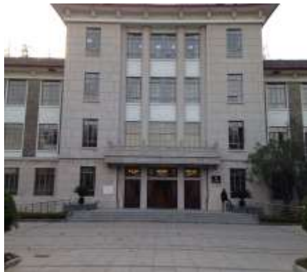
One of three NYU Shanghai buildings: the Library is located in this building. Photographer: Ray Pun.
